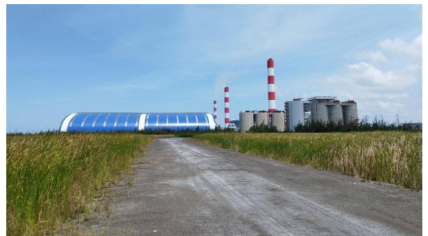
Fig. 7: Using ash and slag to install road base inside Duyen Hai Thermal Power Plant [11]
