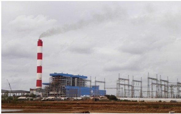
Fig. 1: Duyen Hai 1 Thermal Power Plant [5]
