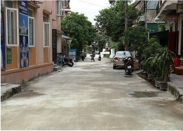
Fig. 12: Urban roads using fly ash and bottom slag materials [30]
