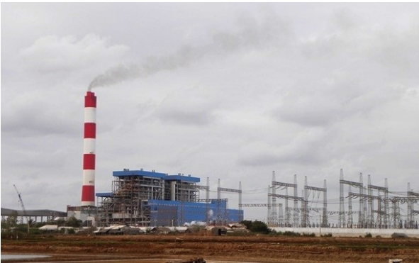
Fig. 1: Duyen Hai 1 Thermal Power Plant [5]
